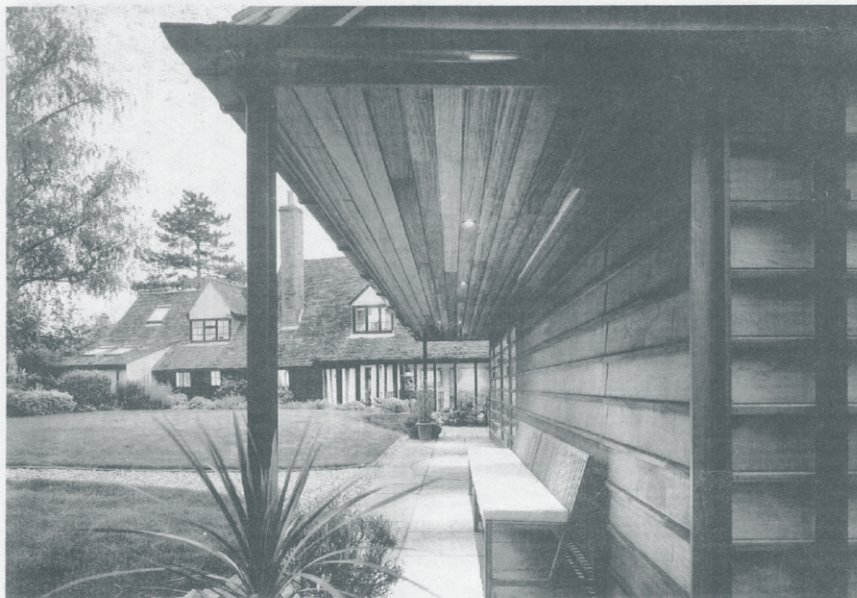
Wood works: the extension is mainly constructed from red cedar ribbed with iroko hardwood
