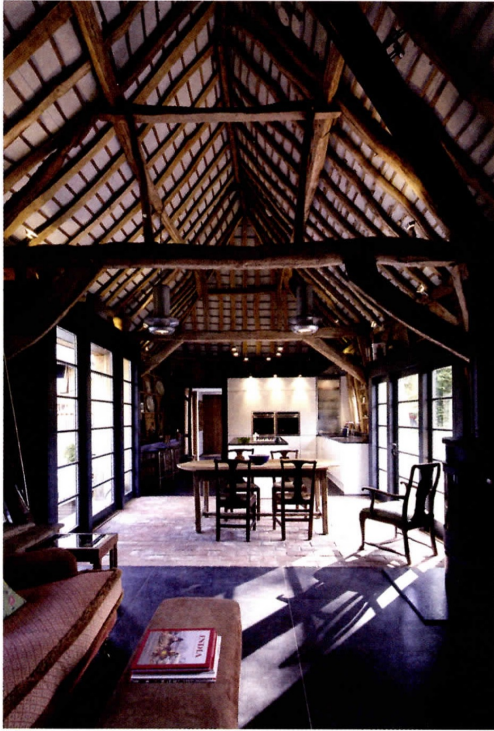
■ The carefully restored structure of the threshing barn
